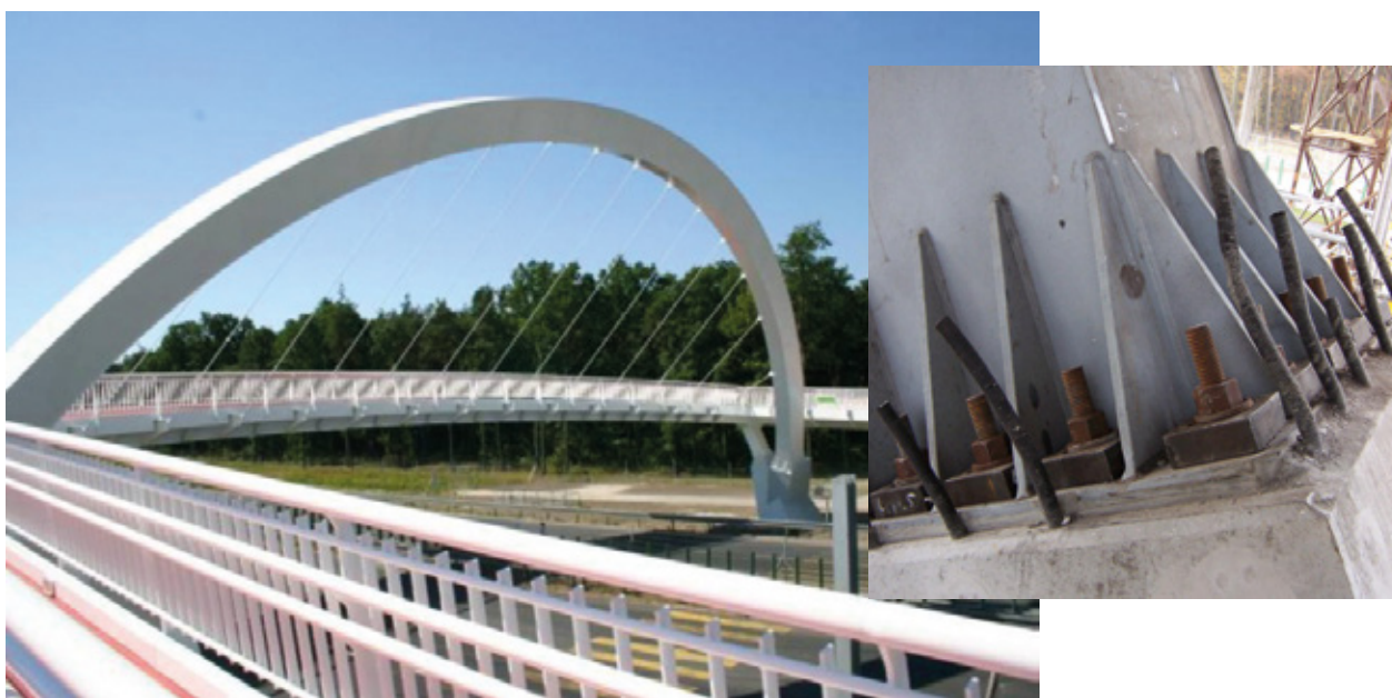
KL8 Footbridge, near Poznan, Poland.
